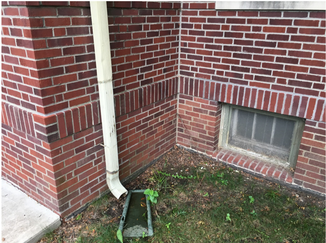
Typical Downspout Emptying On-Grade
