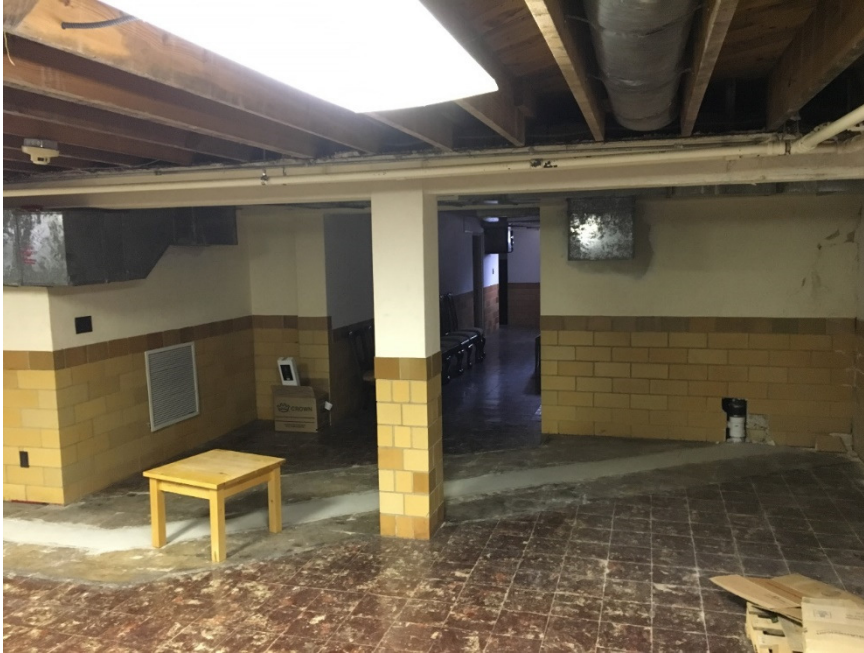
Basement, Recreation Room
