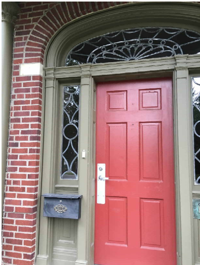
Front Door & Hardware
